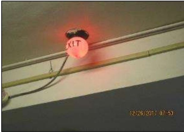
2 nd Floor Hallway.
